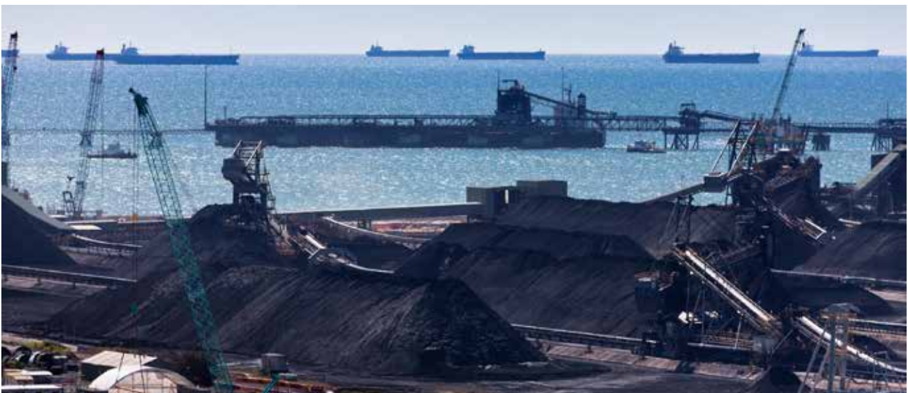
Aerial view of Hay Point coal terminal - One of several that export coal through the Great Barrier Reef. 2012 © Tom Jefferson, Greenpeace
