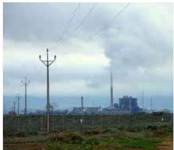
Port Augusta Power station
